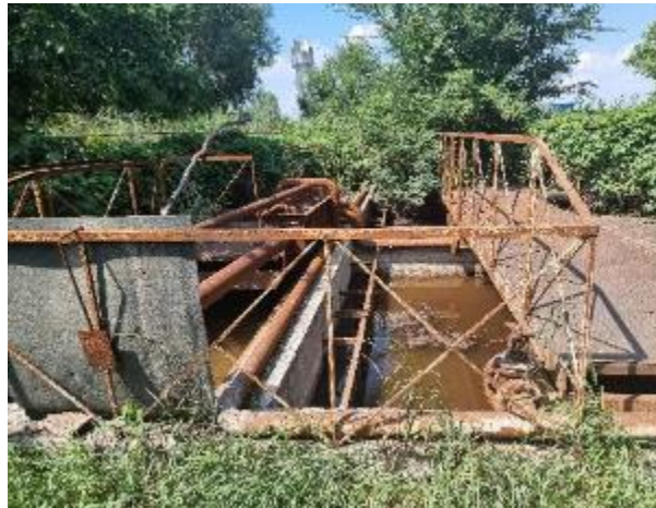
Primary treatment basins, equalization tanks
